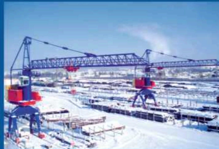
SURGUT, SWL 15 t, 20 cranes
